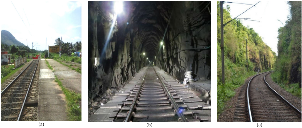
FIGURE 4. OHE at (a) plane ground (b) tunnel (c) earth cuttings.
