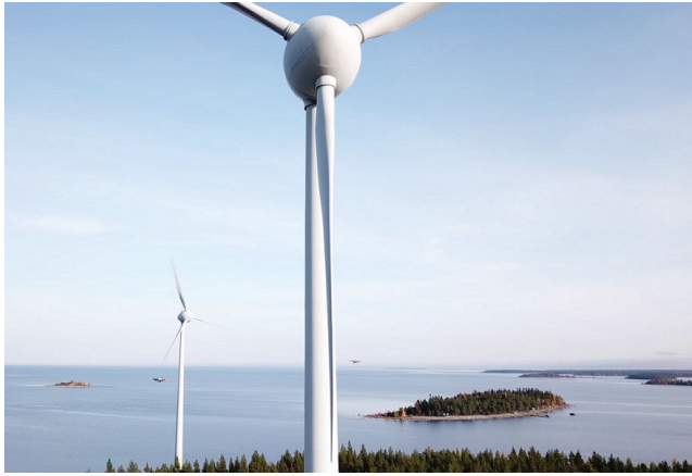
FIGURE 1. The main inspected wind turbine and the MAV, left to the wind turbine in the background, while flying around the blades, where it should be noted the profound scale of the infrastructure in relation to the MAV.
