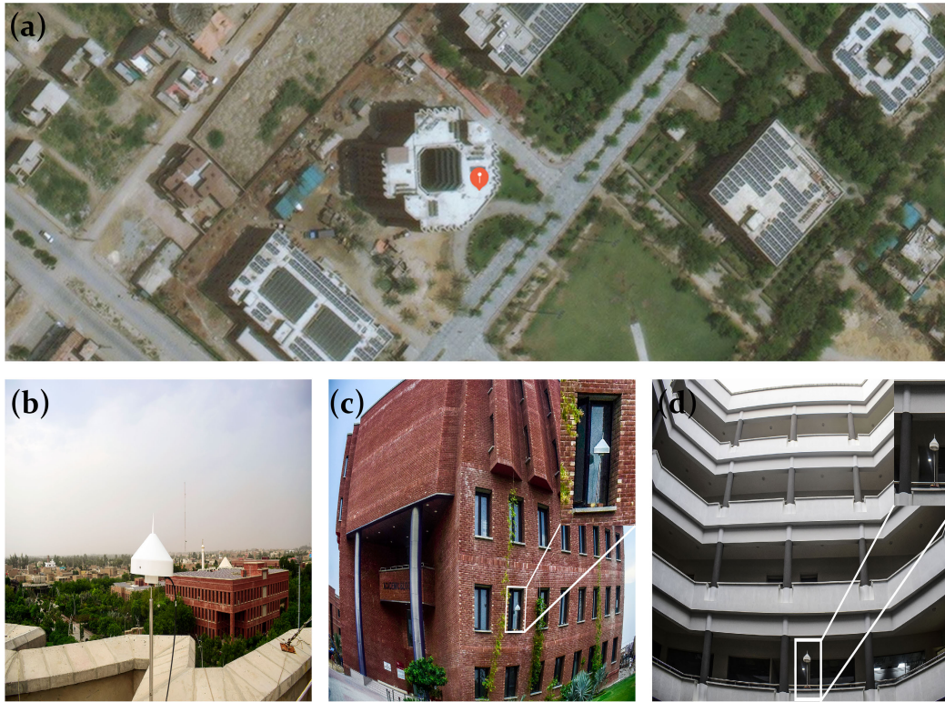
FIGURE 6. (a) Experimental site for single and multi-constellation GNSS data collection. (b) Antenna at the rooftop for clear open sky, (c) Partially degraded environment (Half sky), (d) Highly dynamic multipath environment (Quarter sky).
