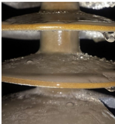
FIGURE 4. Surface hydrophobicity of the insulator units, HC6.
