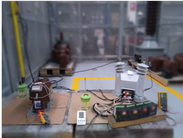
FIGURE 23. Instrument transformer during the heating test.
