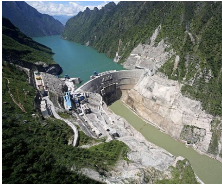
FIGURE 5. Photo of the selected dam.
