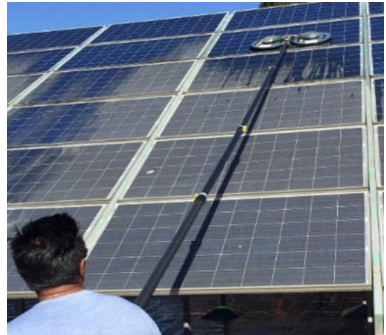
FIGURE 2. Manual hand cleaning system.
