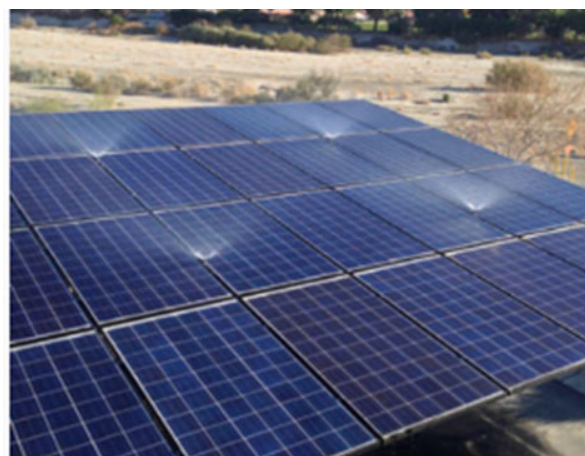
FIGURE 8. Automatic water sprinkler [79].
