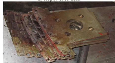
(c)Overheated ablated magnetic pole lamination
