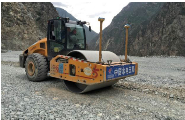
FIGURE 8. Automatic compaction experiment on the main rockfill.
