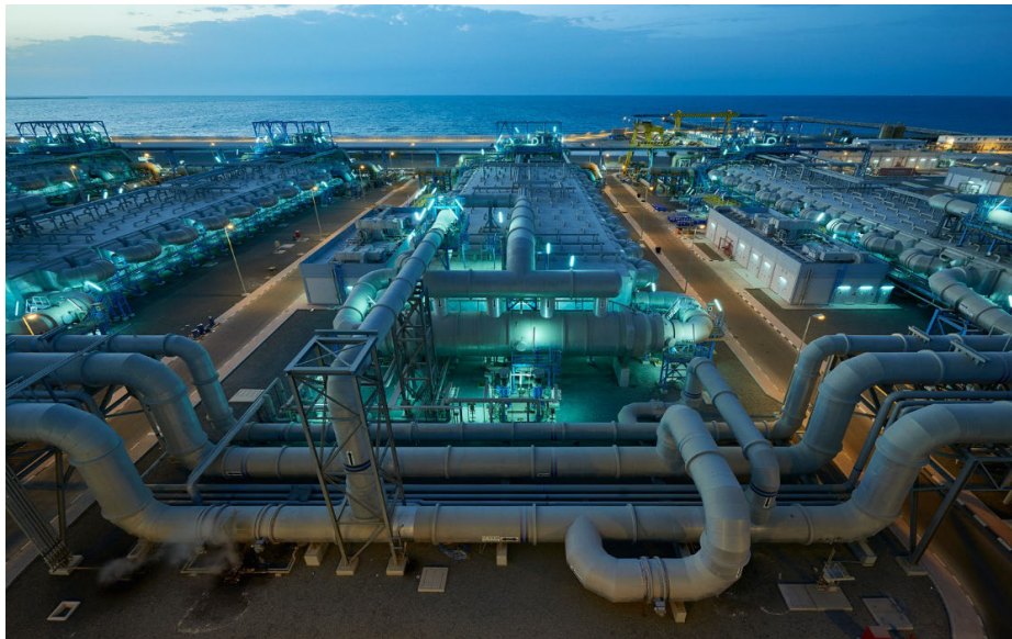
FIGURE 3. Dubai's huge desalination plant [56].
