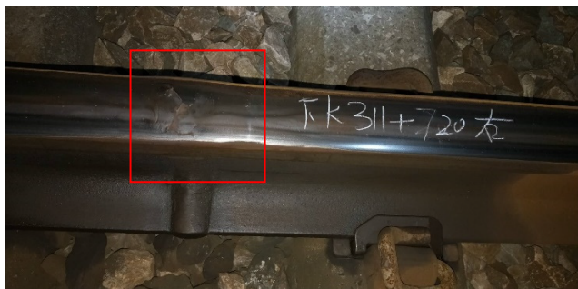
FIGURE 1. Rail weld defects.
