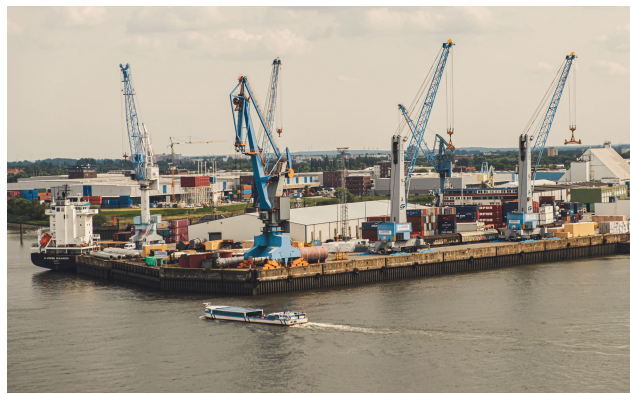
(a) Quay crane. Photo by Moritz Kindler on Unsplash.
