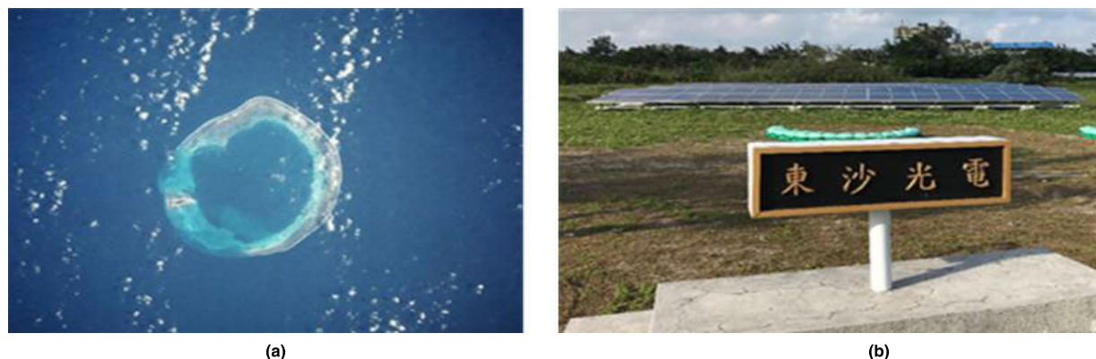
FIGURE 1. Pratas island a) satellite photo and b) existing 40kWp PV system.
