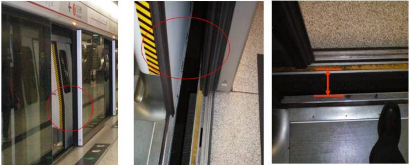
FIGURE 1. The gap between PSD and metro door.
