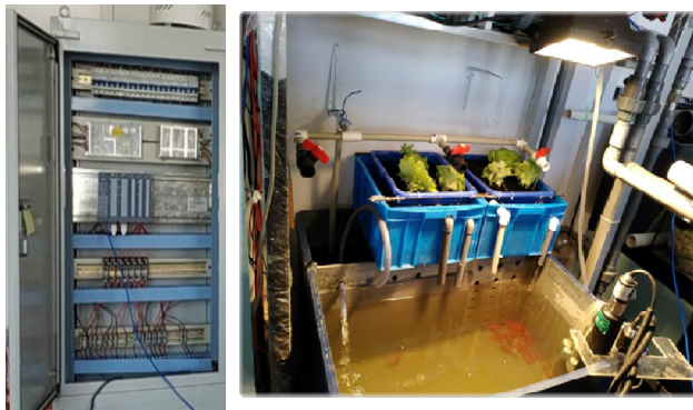
FIGURE 3. Construction of aquaponics system.
