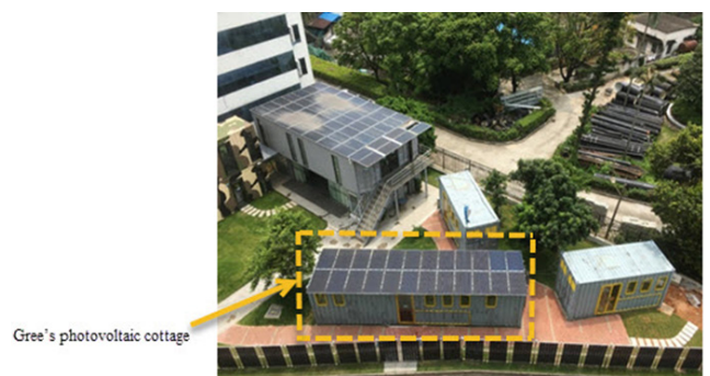
FIGURE 5. Top view of Gree's photovoltaic cottage.
