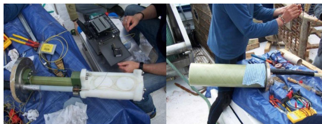
FIGURE 14. Termination box and the optical fiber connection.
