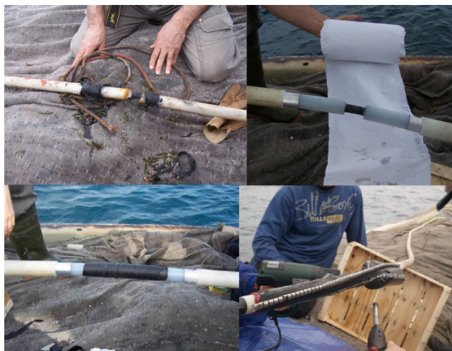
FIGURE 13. The cable before and after the repairs.
