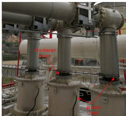
FIGURE 1. GIS enclosure discharge structure diagram.
