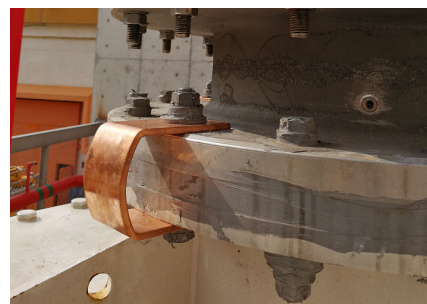
FIGURE 14. Flange layout after bonding.
