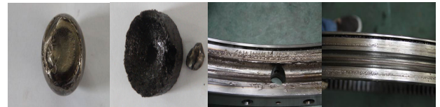
FIGURE 12. The disassembly of the slewing bearing.
