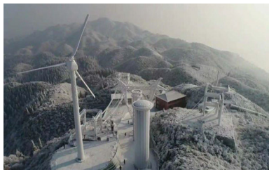
FIGURE 1. Aging environments of composite insulators in a high altitude area experimental station.
