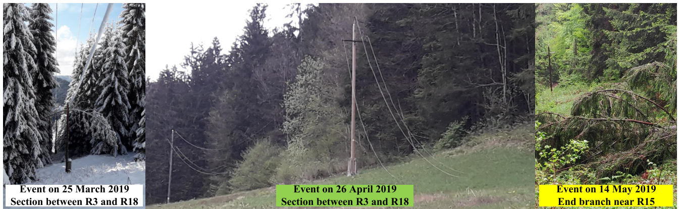
FIGURE 15. Photographs of Ph-Ph faults due to falling trees.
