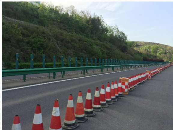
(a) One of two lanes closed on freeway G5
