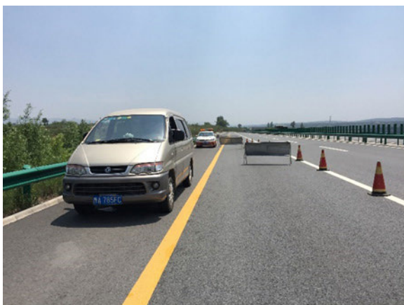
(b) One of three lanes closed on freeway G65
