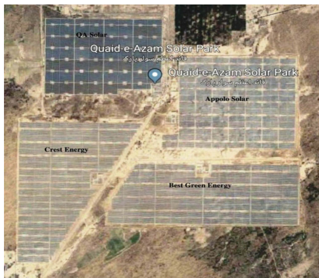
FIGURE 1. Location of the 4 x 100 MW Solar Power Plants in Quaid e Azam Solar Park Bahawalpur, Pakistan.
