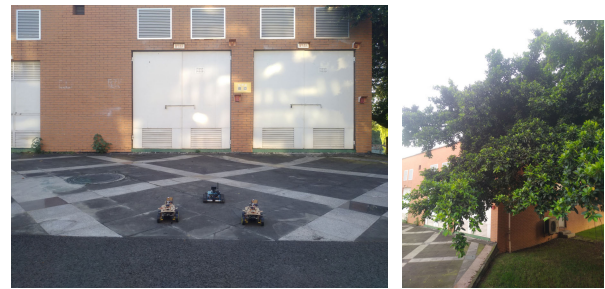
(a) The Monitoring Target – a Voltage Transformer Facility (b) Fixed Camera Monitoring
