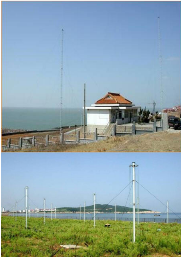
FIGURE 4. Transmitting antenna array and Receiving antenna array.
