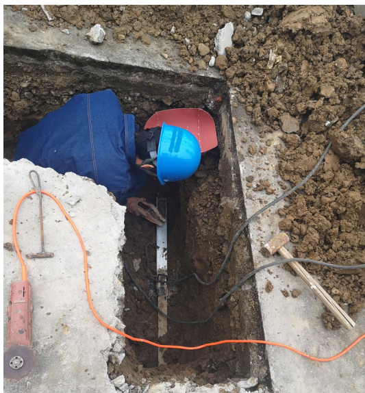
FIGURE 19. Excavation to verify the correctness of result.
