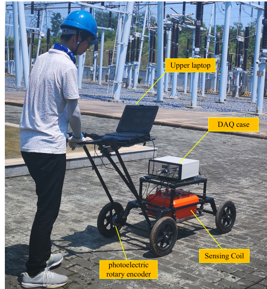
FIGURE 13. A demonstration of NDT equipment for grounding grids.
