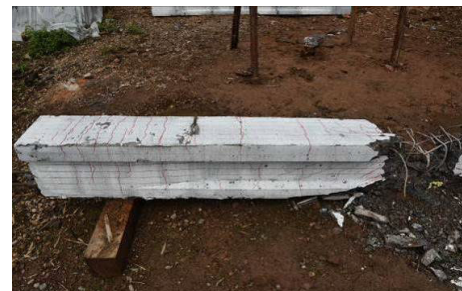
FIGURE 18. Left half span crack distribution of SJ-3.
