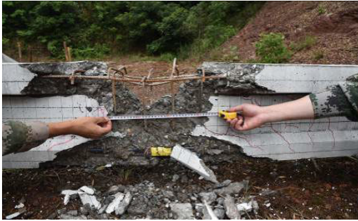
FIGURE 22. Mid-span transverse fracture of SJ-2.
