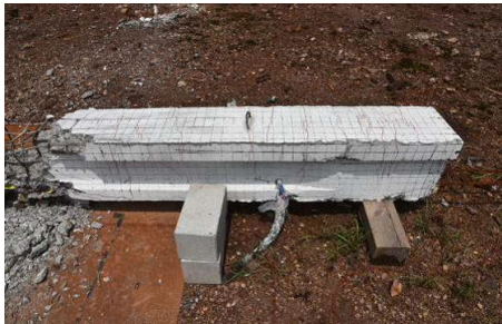
FIGURE 15. Right half span crack distribution of SJ-1.
