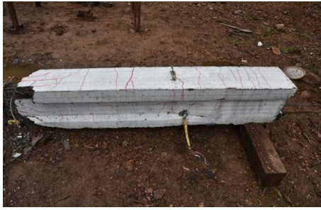
FIGURE 19. Right half span crack distribution of SJ-3.
