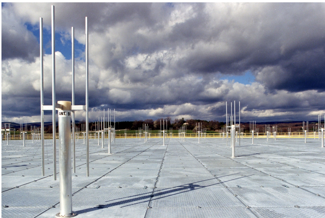
FIGURE 2. Photography of the sparse receiving array.
