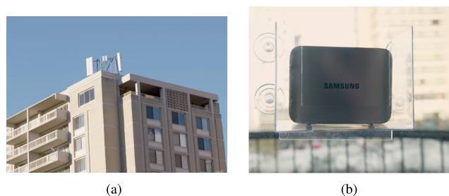
FIGURE 8. (a) Verizon 5G infrastructure (smallcell) on roof, and (b) Samsung home unit (femtocell) attached on window [42].
