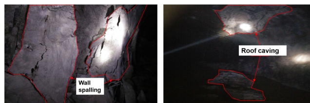
FIGURE 2. Roadway damage caused by high shearing stress.
