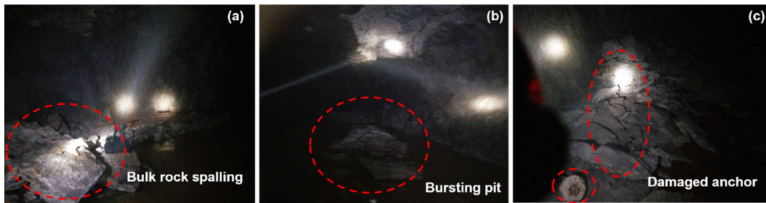
FIGURE 20. Photos of the rockburst accident.
