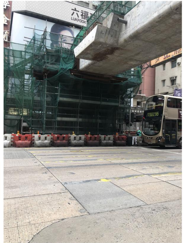
**FIGURE 7.** Upgrading of at-grade pedestrian crossing to a grade-separated flyover.
