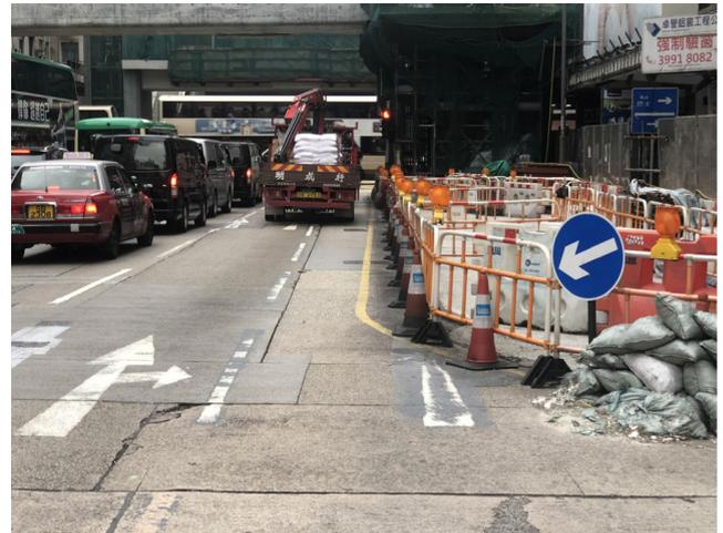
FIGURE 5. Alterations of existing lane markings due to temporary roadworks.
