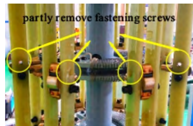
b. Simulating the loosening of moving contact
