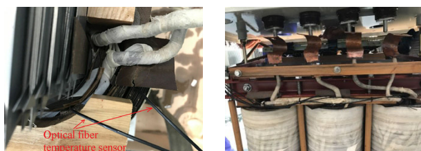
FIGURE 3. Optical fiber temperature sensors arrangement in temperature rise test.
