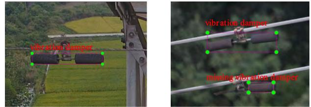
**FIGURE 11. Vibration damper detection.**
