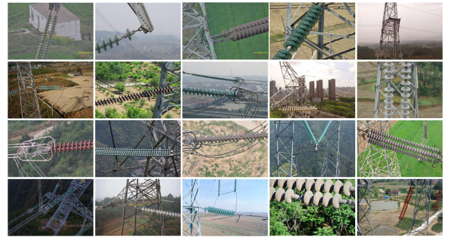
FIGURE 6. Samples of collected aerial images including varied insulators with complex backgrounds.
