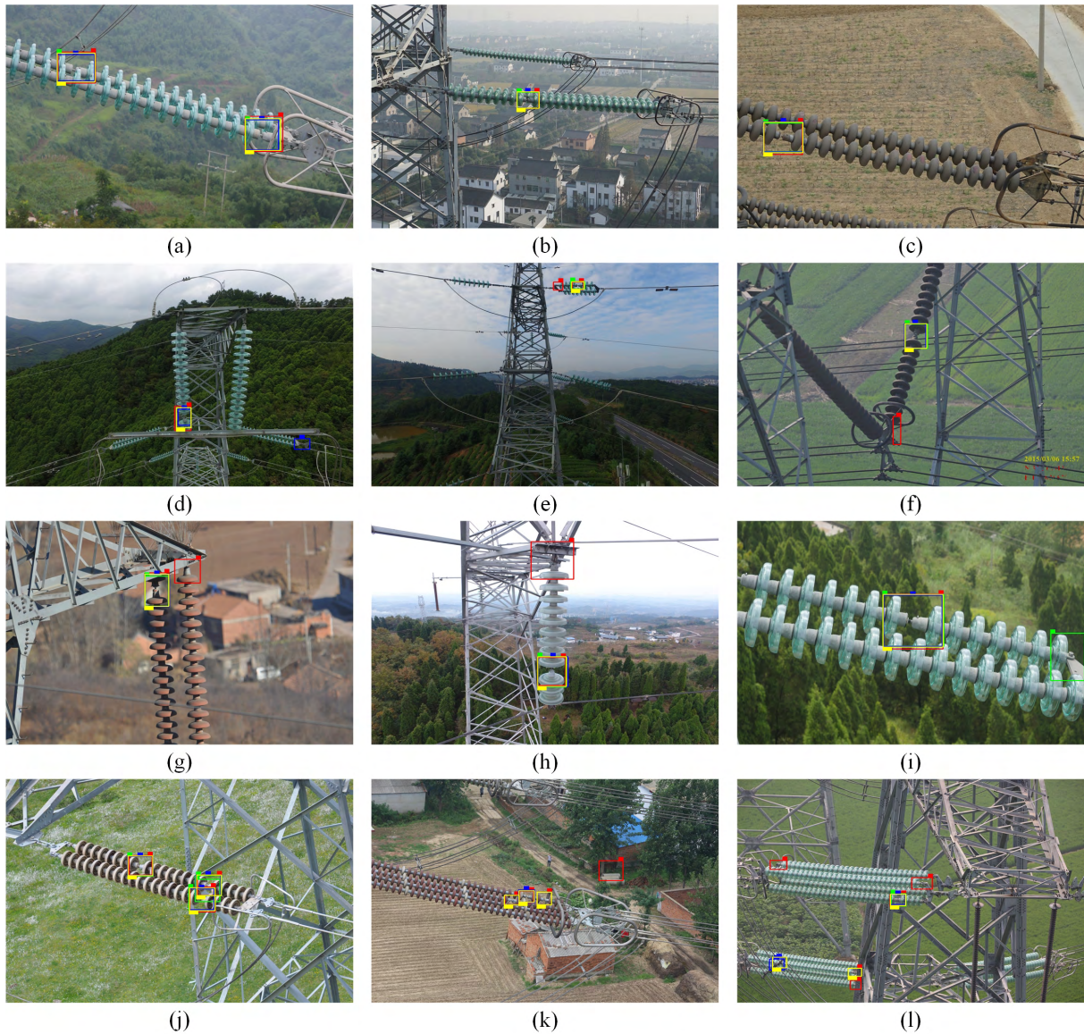
FIGURE 12. Comparison between single-level perceptions and multi-level perception. The green, blue, and red boxes denote the results of low level, middle level, and high level respectively. Results of multi-level perception are bounded by the yellow box.
