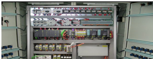
FIGURE 9. Power transformer detection panel developed in Mersin University Laboratory.
