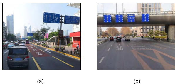
FIGURE 2. Offset transit lane used in Shanghai and Dalian. (a) Xizang Nanlu (Shanghai) and (b) Gao'erji Lu (Dalian).
