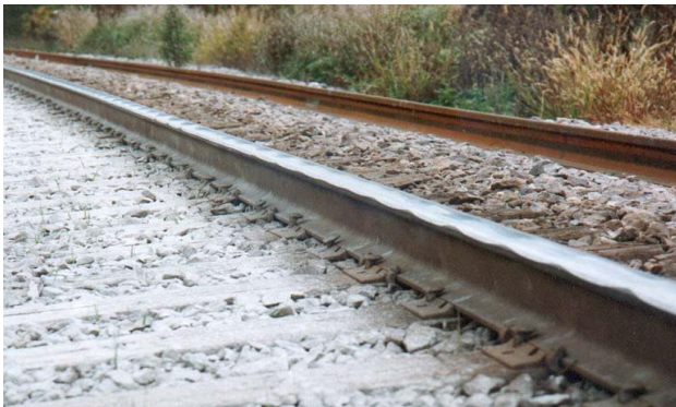
FIGURE 2. Irregularities on rail surfaces.
