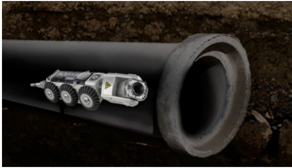
FIGURE 2. CCTV Inspection (Image from M. TUCKER & SONS).
