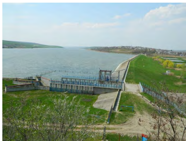
FIGURE 2. Drăcșani dam and artificial lake © http://www.visitbotosani.ro/ .
