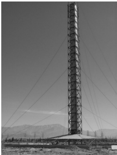
FIGURE 1. Kerman pilot solar chimney power plant.
