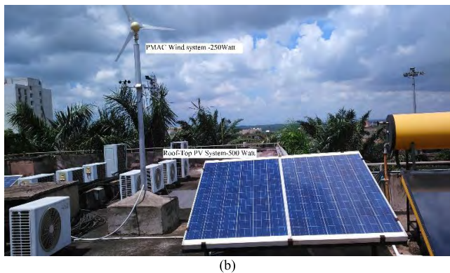
FIGURE 23. (a) Experimental Set Up for hardware realization, (b) Roof-top PV and wind system.
