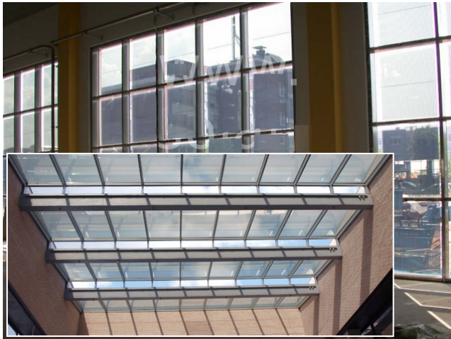
FIGURE 1. Building Integrated Photovoltaic.
