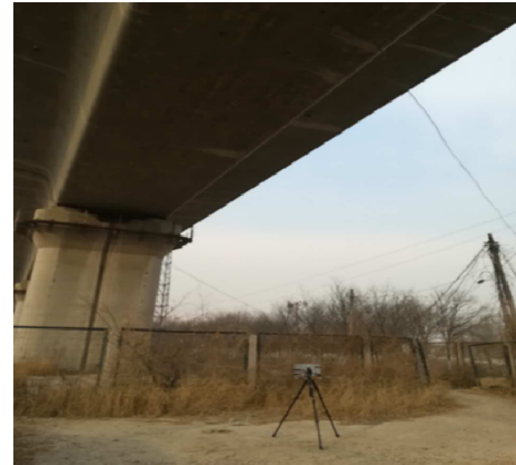
FIGURE 5. Experiment setup of the high-speed railway bridge.
