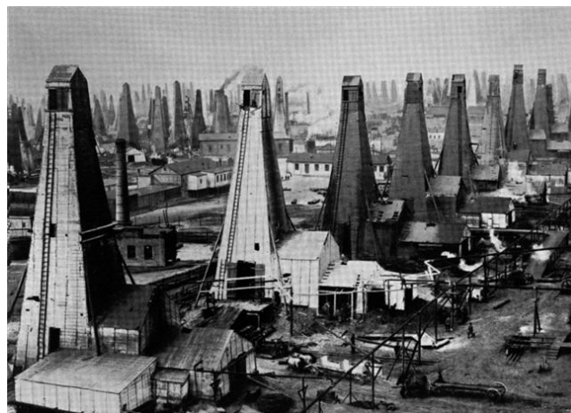
FIGURE 7. The Branobel Company of the Nobel brothers owned the oil derricks in the Balachany field (near Baku, Azerbaijan, end of the nineteenth century). At that time, drilling was mainly devoted to producing kerosene for lighting, and the size of the plants suggest the economical relevance of the enterprise. (Photo courtesy of Tekniska Museet on Wikimedia Commons).
