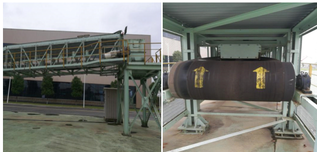
FIGURE 7. Testing on power balance of pipe belt conveyor.
