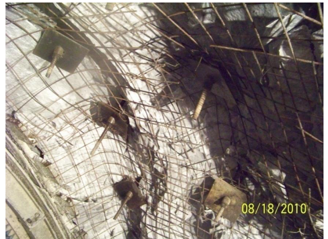
FIGURE 6. Photograph of the intense rockburst which occurred at chainage K10+4350–356 on 18 August 2010.
