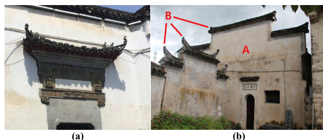
FIGURE 3. Typical decorations of Huizhou architecture: (a) gatehouse; (b) white wall, which is indicated by A, and Mar tau wall (top component of the white wall, also known as horse-head wall), which is indicated by B.
