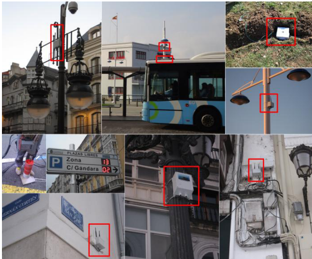
FIGURE 1. Real SmartSantander deployment examples.
