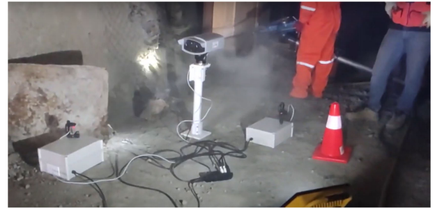
FIGURE 16. Underground tunnel under extreme dust conditions.
